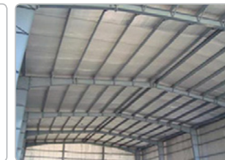
Roof insulation
